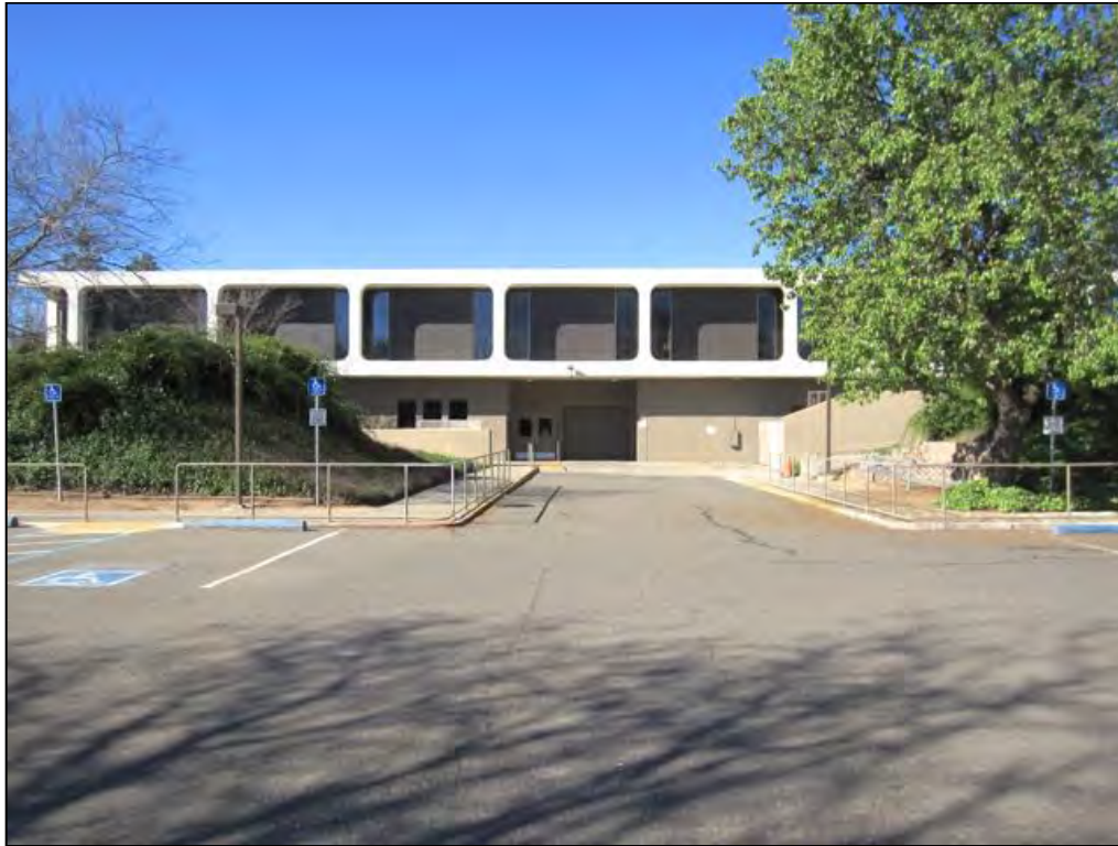
Figure 13: Photograph of east façade, camera facing west, 1 March 2015.
