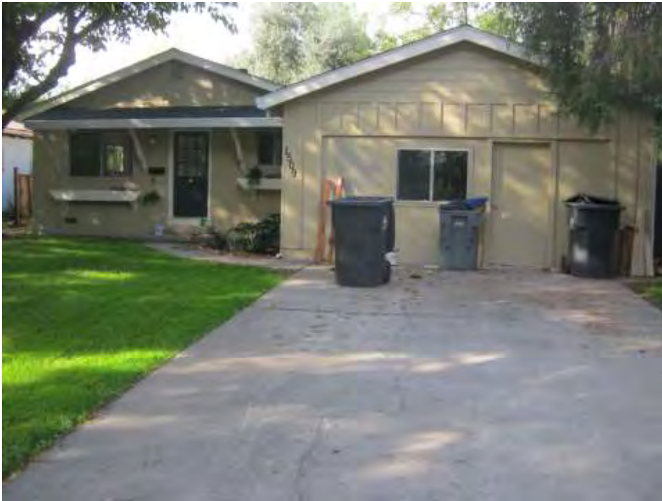
Photograph 9: Heavily altered house at 1509 Cypress Lane, 1962.
