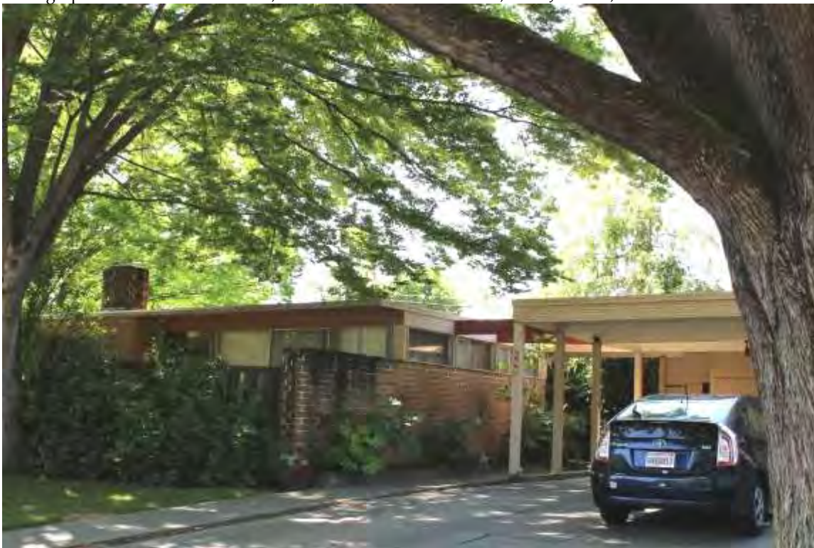
Photograph 14: 658 Elmwood Drive, east elevation, camera facing southwest, designer unknown, 1958.
