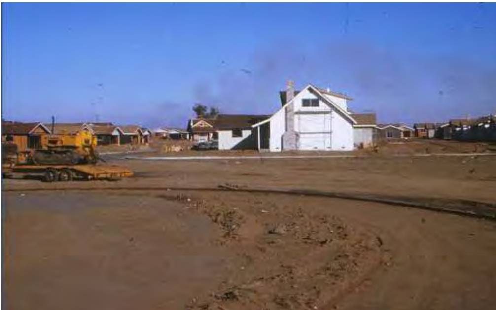
Figure 14: Grinnell Drive under construction, 1972 (courtesy John Lofland).
