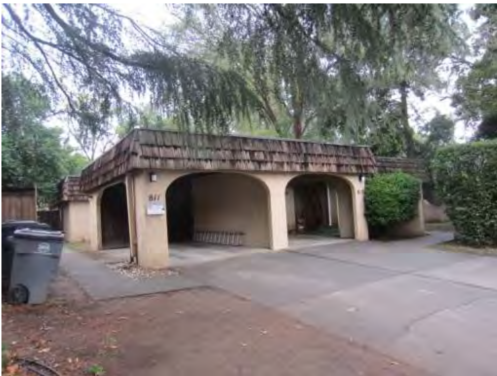
Photograph 4: 811 & 813 Arthur Street, Example of moderately altered Mansard style duplex, 1972.
