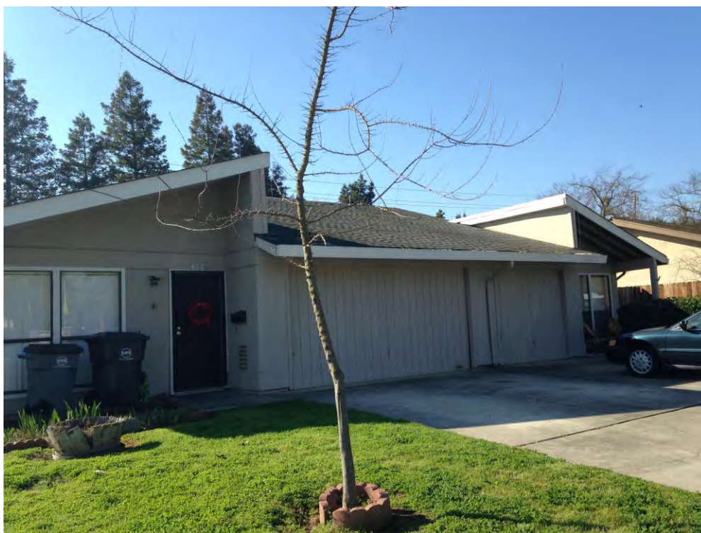
Photograph 2: 4718 and 4720 Cowell Boulevard, Example of duplex with two shed roofs, 1973.
