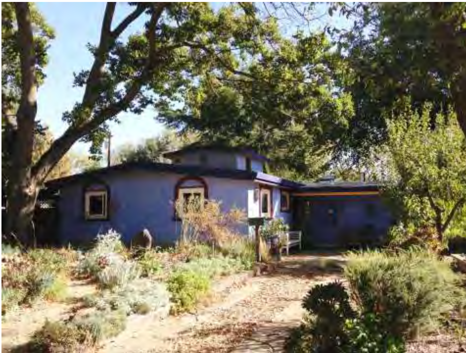
Photograph 5: Heavily altered house with garage conversion, second story addition, stucco cladding and other changes at 704 M Street, 1956.
