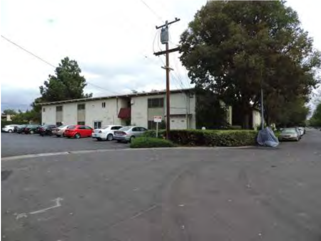
Photograph 1: 911 Pennsylvania Place, Large 2-story apartment building with flat roof, 1966.
