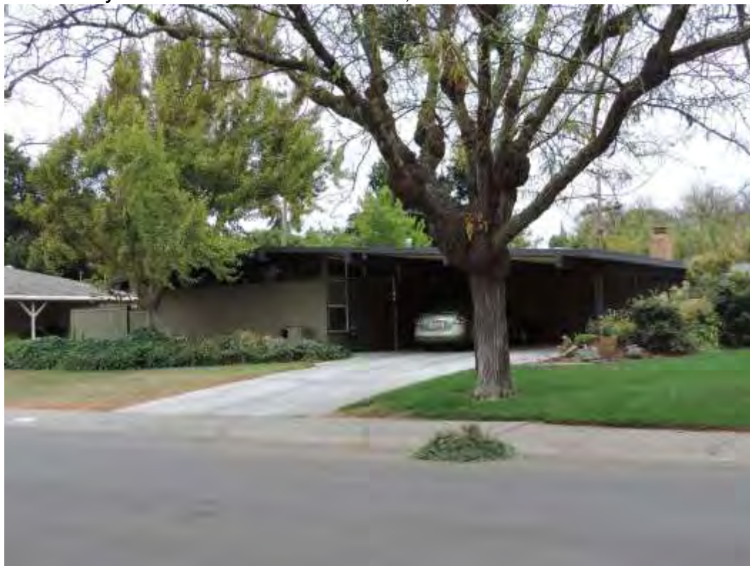
Photograph 3: 1144 Princeton Place, Example of moderately altered Post-and-Beam "Classic" with double carport, 1963.
