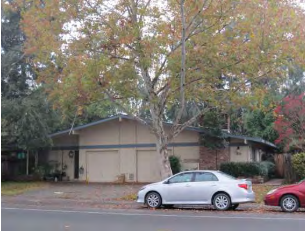
Photograph 5: 817 & 819 Arthur Street, Example of moderately altered L-shaped duplex with gabled roof, 1971.
