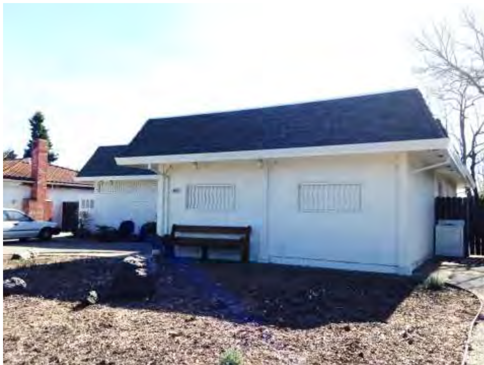
Photograph 1: 3620 Chiles Road, Example of moderately altered L-shaped house with mansard roof, 1966.
