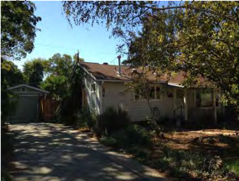
Photograph 4: 806 Eleventh Street, Moderately altered Minimal Traditional house.
