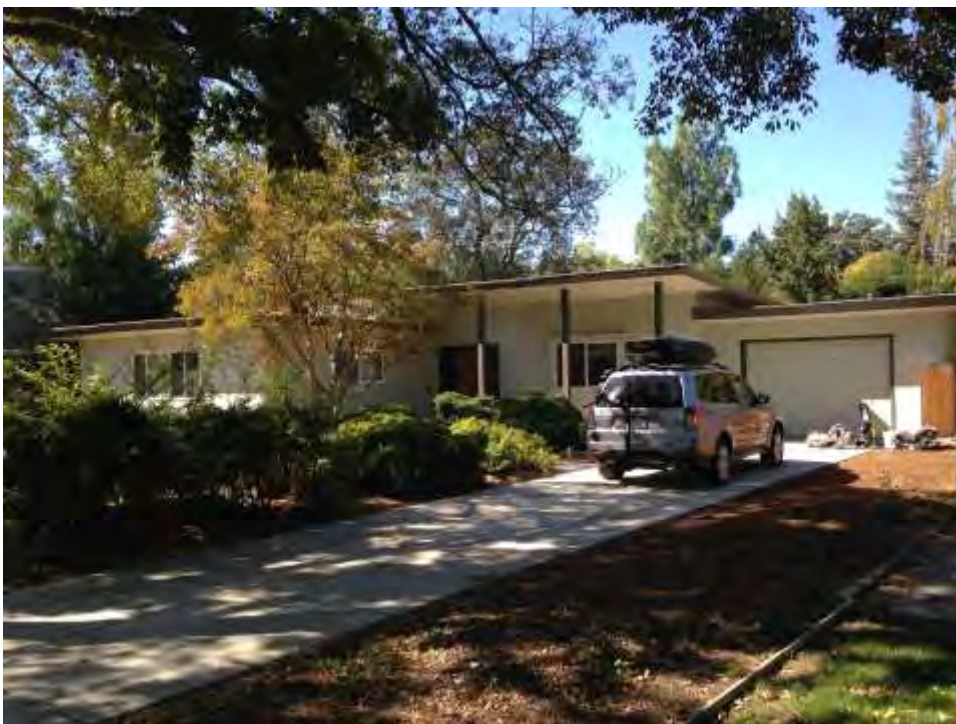
Photograph 6: Heavily altered flat-roofed Contemporary house at 5 Parkside Drive, 1951.
