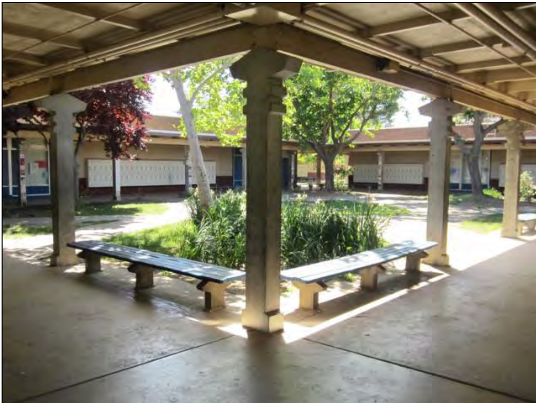
Figure 5: Cast concrete columns at Holmes Junior High School. Photograph 19 April 2015.
