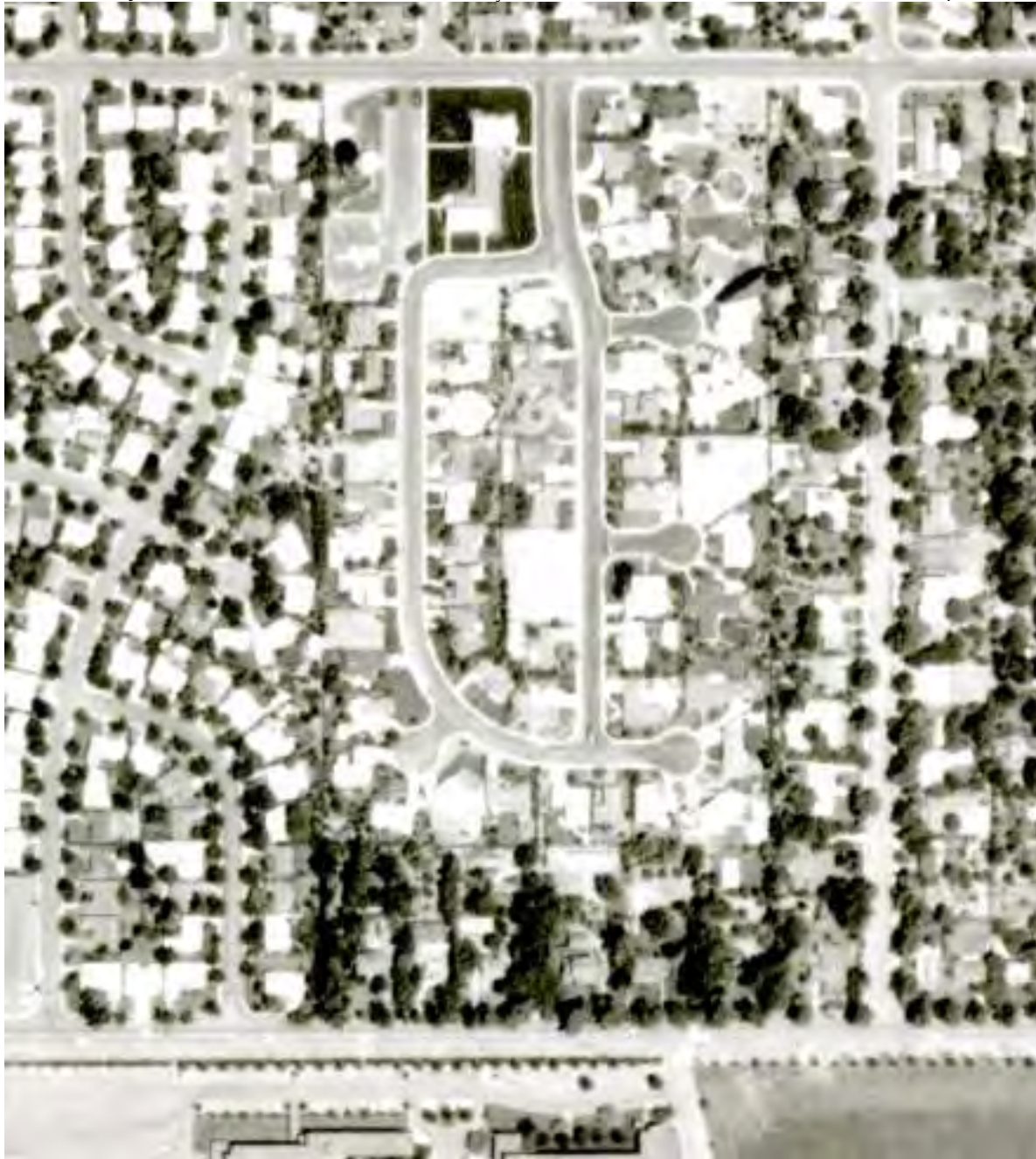
Figure 4: U.S.D.A. Aerial Photograph of Elmwood Subdivision, 1964. Most lots were developed at this point.
