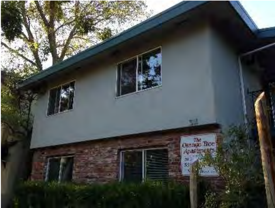
Photograph 5: 311 Seventh Street, Small two-story apartment building.
