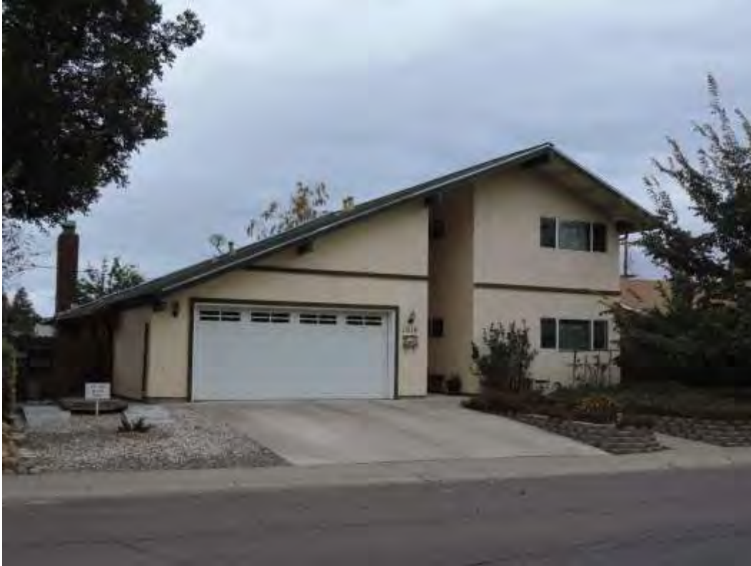
Photograph 12: 1019 Alice Street, Example of heavily altered 2-story house, 1965.
