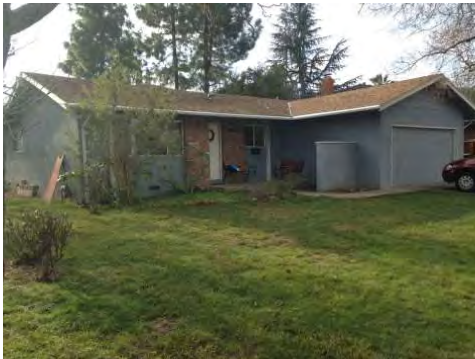
Photograph 1: Moderately altered gabled Tract Ranch with decorative beams at 422 Cabrillo Avenue, 1970.
