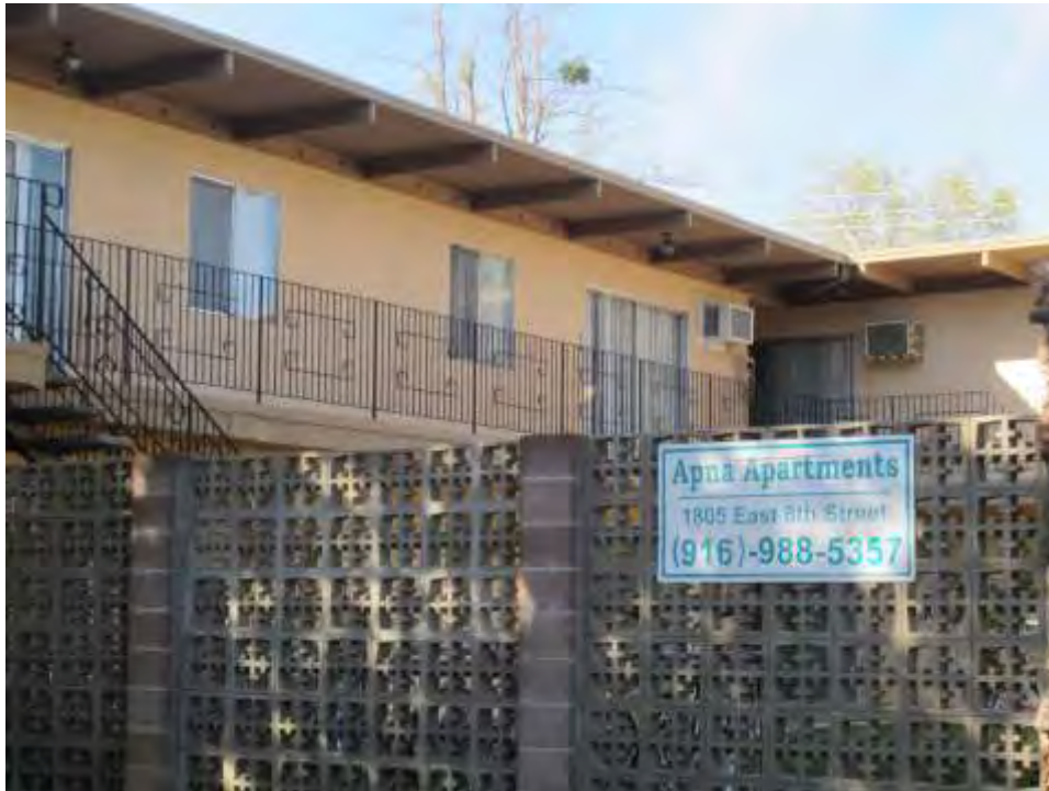
Photograph 13: Moderately altered two-story Apartment Building at 1805 East Eighth Street, 1964.
