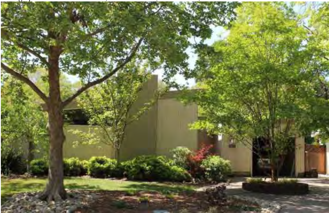
Photograph 10: 638 Elmwood Drive, east elevation, Gale Sosnick, 1958.
