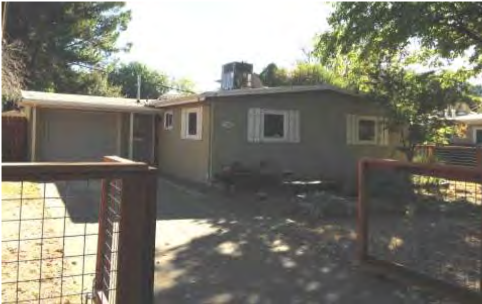
Photograph 2: Moderately altered Tract Ranch house at 708 L Street, 1955.
