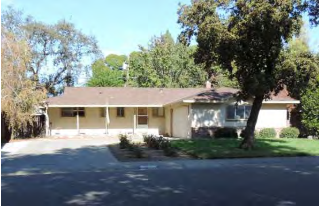
Photograph 6: 1507 Alice Street, Example of moderately altered L-shaped Ranch house with hipped roof, side-entry garage with metal replacement door, and original horizontal aluminum slider windows.
