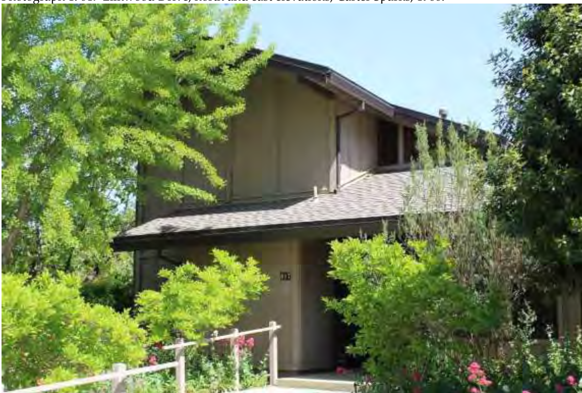
Photograph 2: 617 Elmwood Drive, west elevation, Carter Sparks, 1966.
