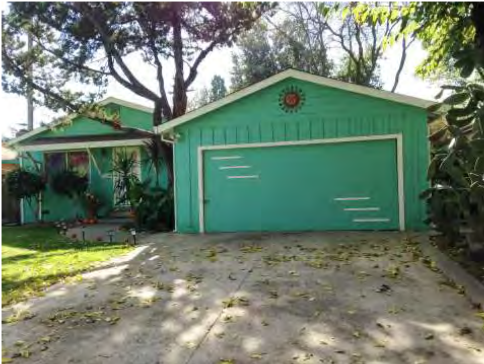
Photograph 7: Moderately altered shed roof porch Tract Ranch at 1712 Albion Place, 1961.
