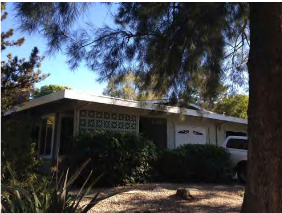
Photograph 6: 537 & 539 Scripps Drive, Example of moderately altered Contemporary duplex with concrete screen wall, 1969.
