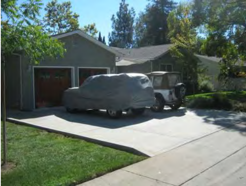
Photograph 1: U-shaped Ranch house at 39 Parkside Drive, 1951.
