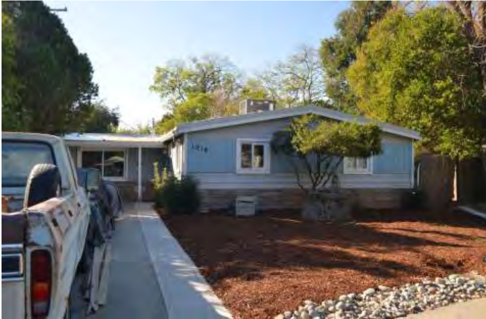
Photograph 4: Heavily altered house with garage conversion at 1210 Covell Place, 1954.
