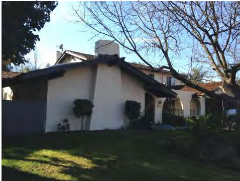
Photograph 7: Moderately altered Spanish Ranch house at 2219 Anza Avenue, 1970.
