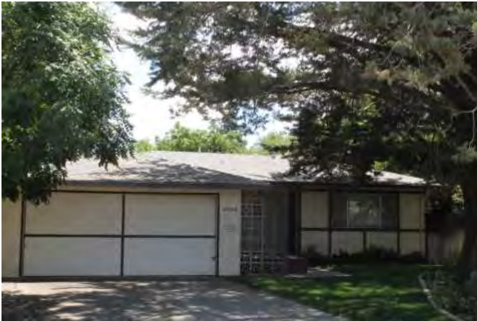
Photograph 2: Unaltered L-shaped house with concrete block screen wall at 2508 Clemson Drive, 1965.
