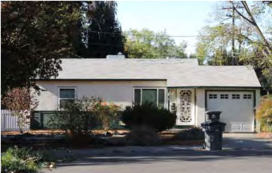
Photograph 3: 9 Simmons Street, Example of moderately altered side-gabled Minimal Traditional house with vinyl replacement windows, and single garage with metal replacement door.
