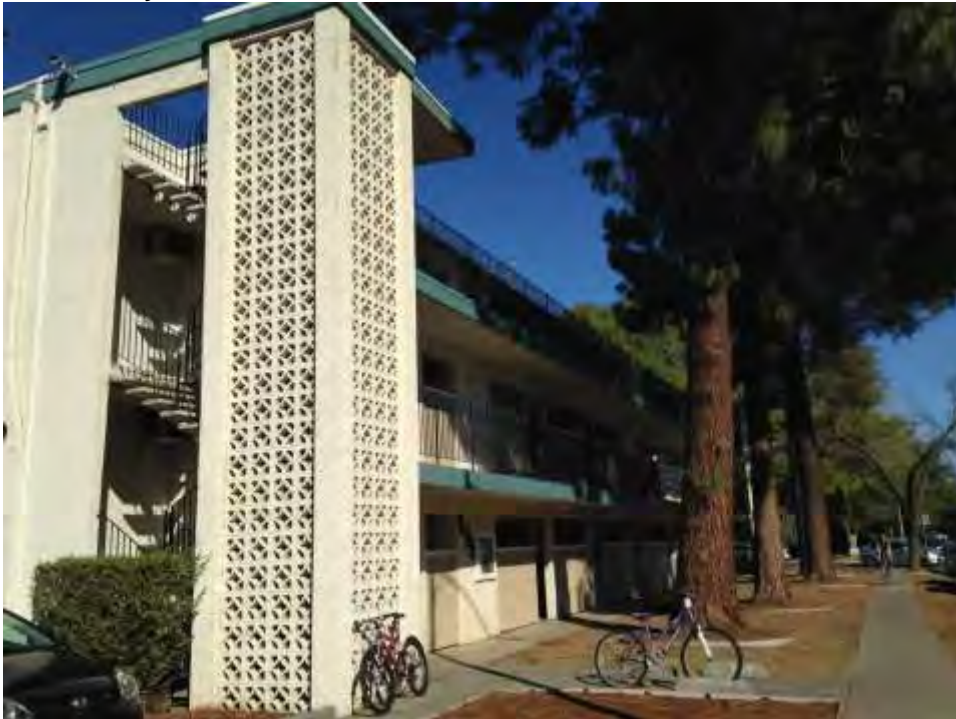
Photograph 9: 835 F Street, Large three-story apartment building with decorative concrete block screen, 1965.
