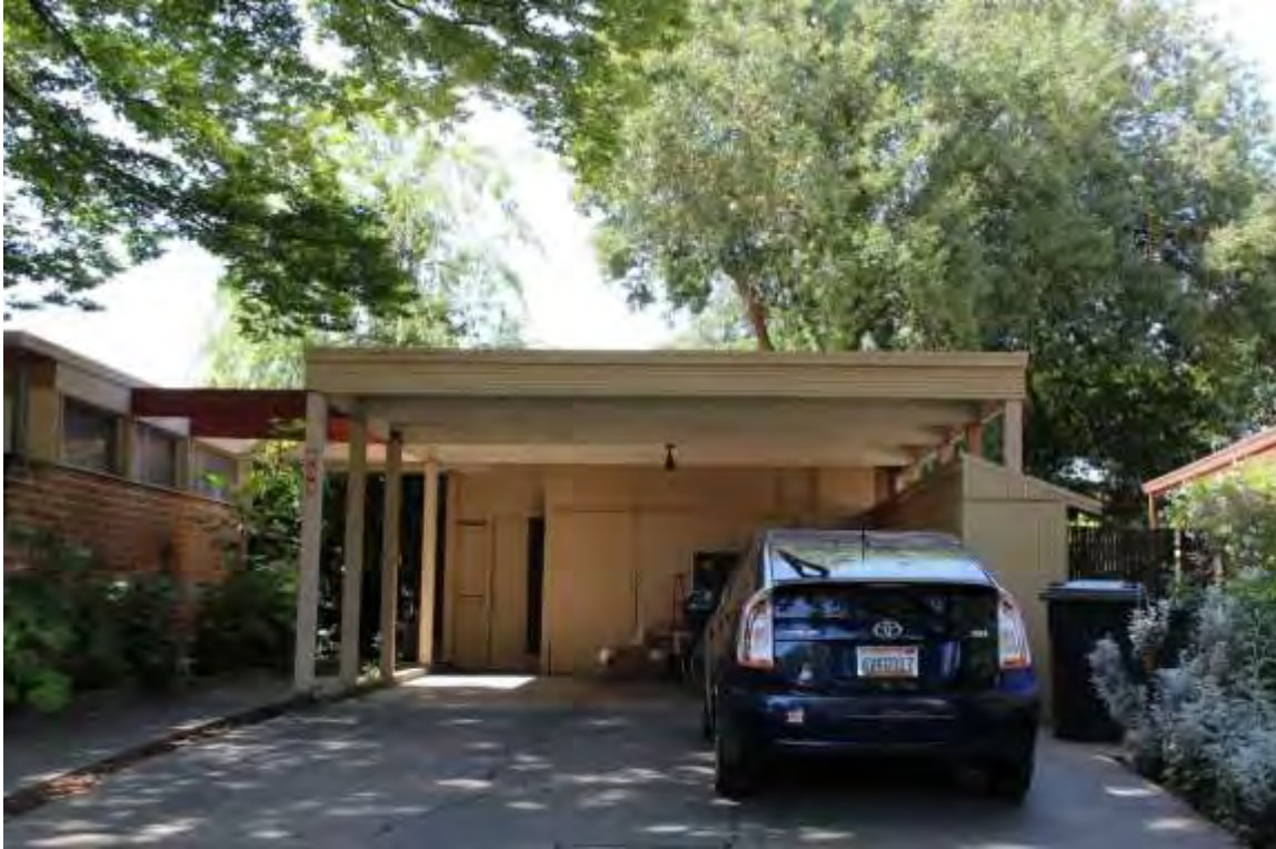
Photograph 15: 658 Elmwood Drive, east elevation showing flat-roofed carport, designer unknown, 1958.
