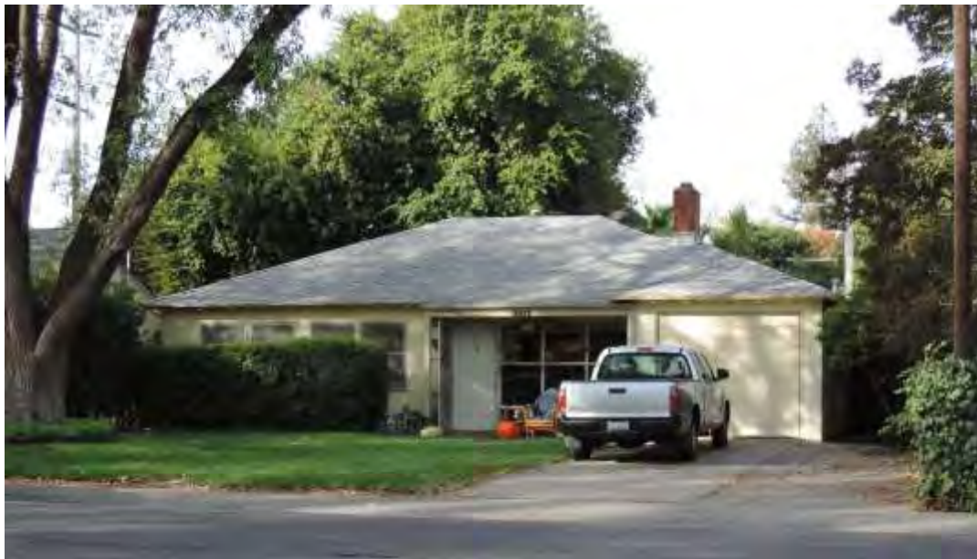
Photograph 1: 853 L Street, Example of unaltered hipped-roof Minimal Traditional house with multiple-light picture window, double-hung wood sash windows, and single garage with wooden door.
