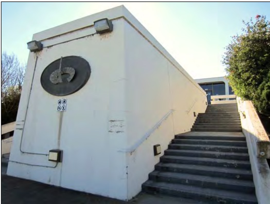
Figure 12: Photograph of building promontory, camera facing southeast, 1 March 2015.
