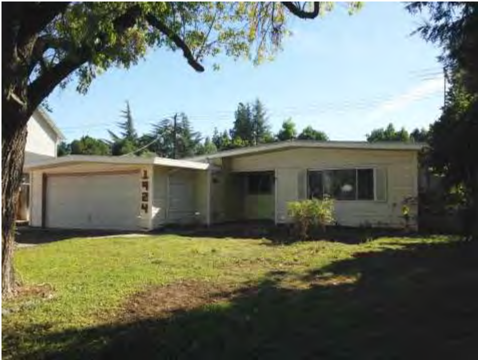
Photograph 3: Moderately altered Tract Ranch house at 1924 Haussler Drive, 1959
