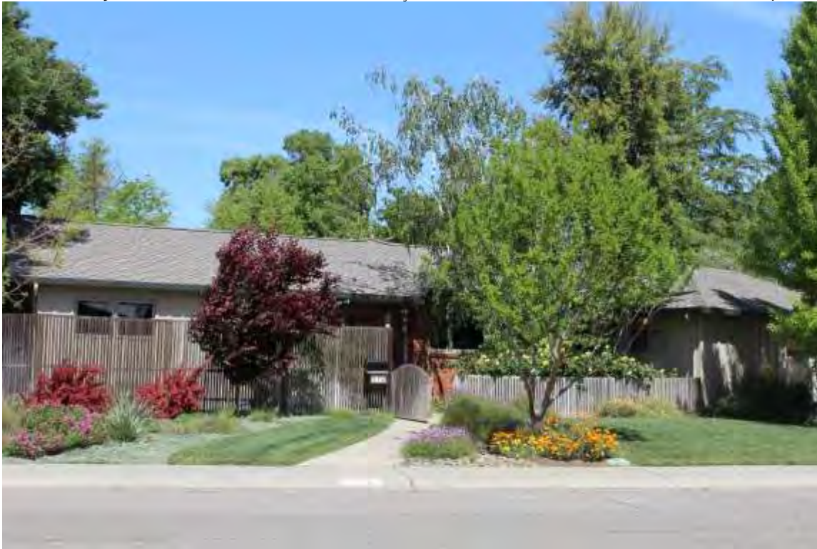
Photograph 46: 776 Elmwood Drive, south elevation, designer unknown, 1958.
