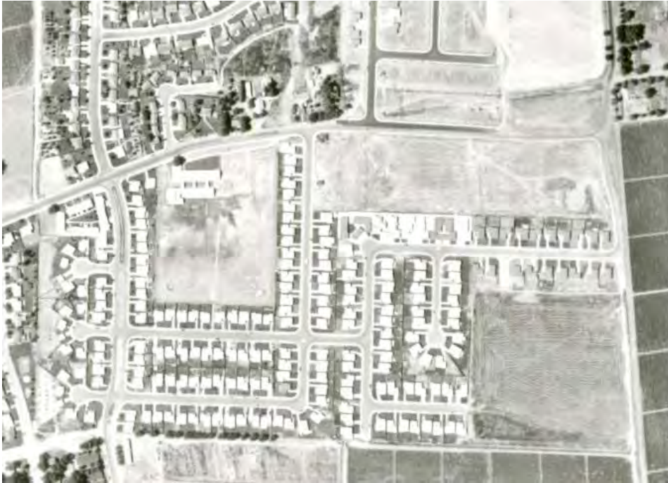
Figure 9: U.S.D.A. Aerial photo showing residential portions of Davis Manor 1 – 6 complete and first elementary school buildings constructed, 1957. East Eighth Street has been straightened, and Davis Manor 7 is under construction.
