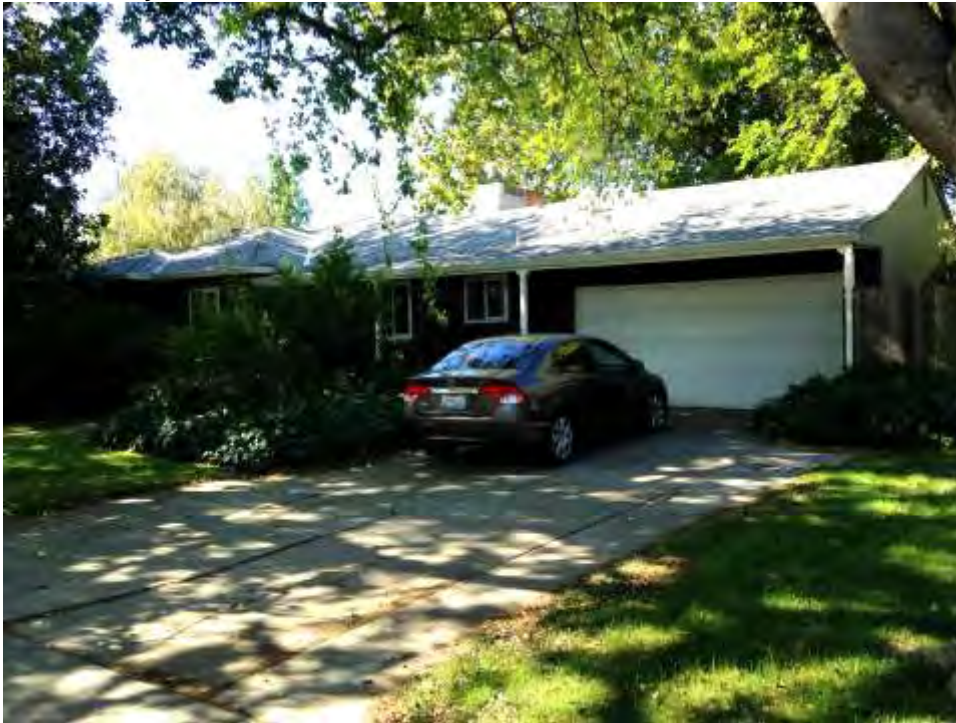
Photograph 3: Heavily altered Minimal Traditional house at 9 Parkside Drive, 1952.
