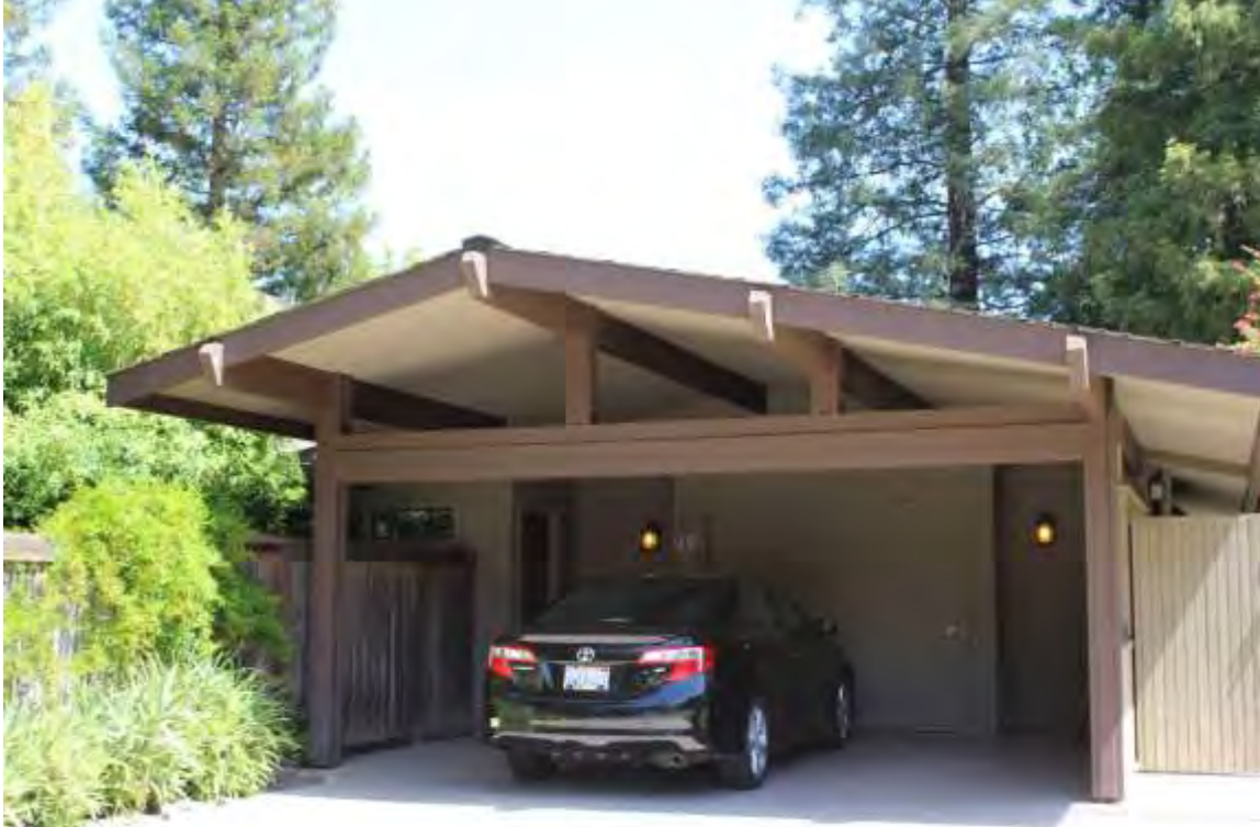
Photograph 29: 732 Elmwood Drive, west elevation, camera facing east, Jim Adams, 1932.
