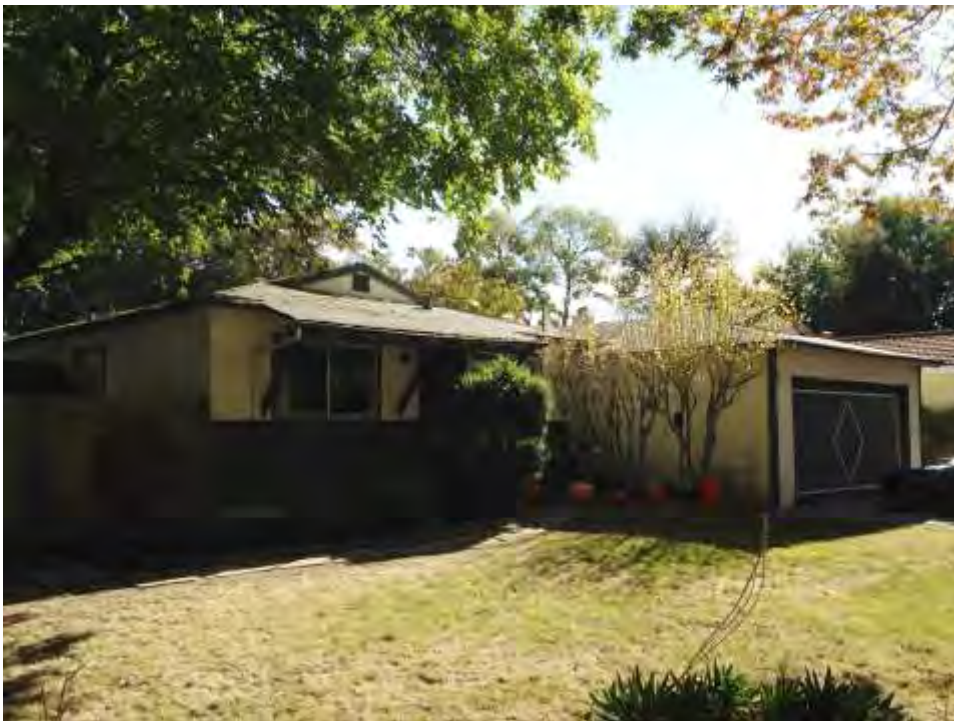
Photograph 6: Unaltered shed porch Tract Ranch at 1712 Madrone Lane, 1961.
