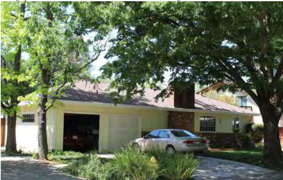
Photograph 8: 634 Elmwood Drive, south and east elevations, John Whitcombe, 1960.
