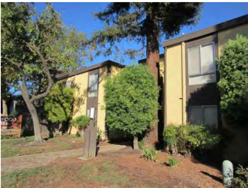
Photograph 10: 607 East Eighth Street, Two-story apartment building, 1973.
