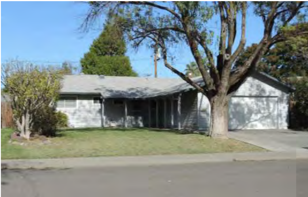
Photograph 5: 1408 Alice Street, Example of moderately altered L-shaped Ranch house with cross-gabled roof, metal replacement garage door, and vinyl replacement windows.
