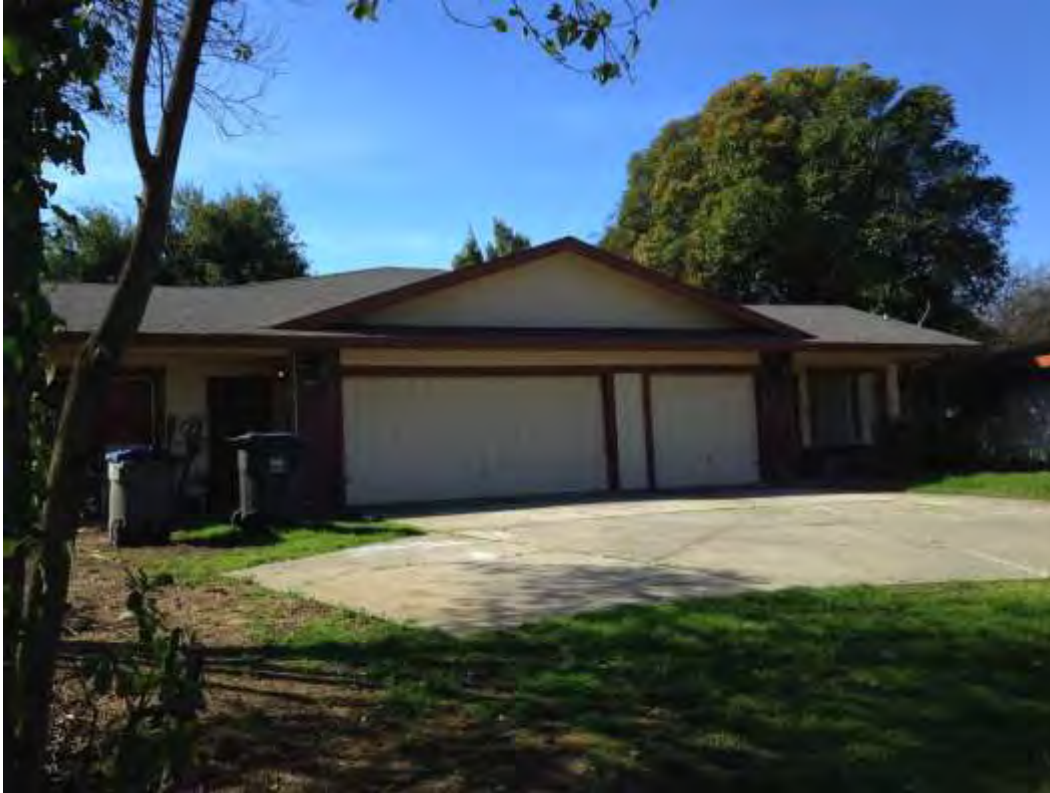
Photograph 3: 217 & 219 La Vida Way, Example of moderately altered linear duplex with cross gabled roof, 1972.
