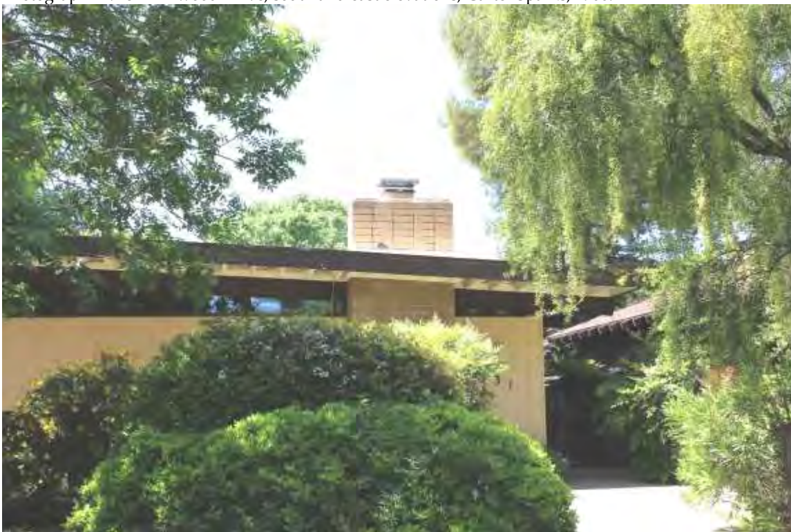
Photograph 28: 731 Elmwood Drive, east elevation, Carter Sparks, 1966.
