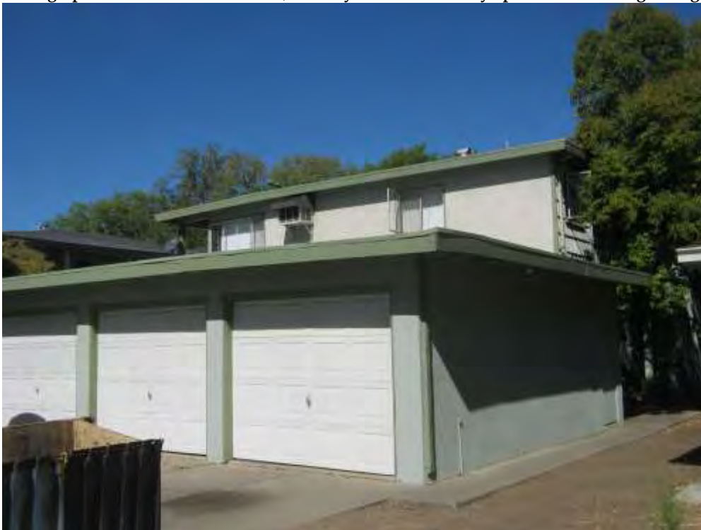
Photograph 2: 803 – 809 Tenth Street, Moderately altered two-story apartment building with ground-floor garages.
