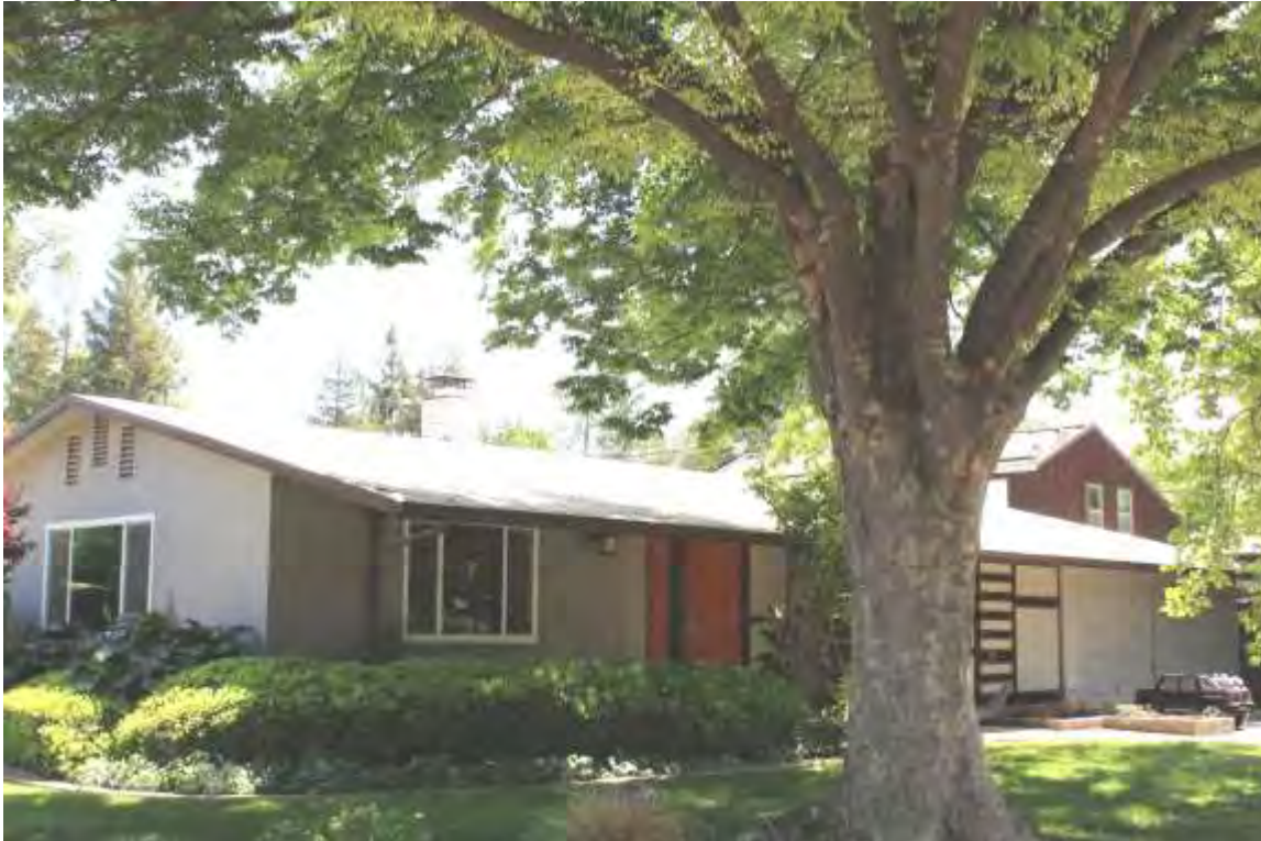
Photograph 41: 760 Elmwood Drive, north and west elevations, designer unknown, 1959.
