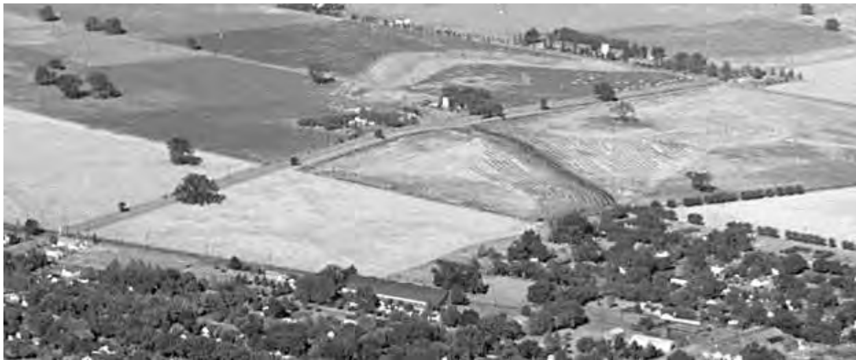
Figure 3: Oblique aerial photograph of Huntwood Park area, 1946.
