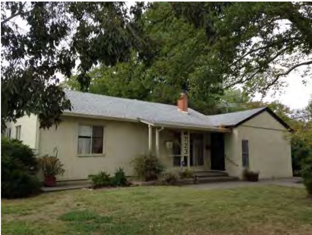
Photograph 6: 723 J Street, Example of heavily altered Minimal Traditional house with gabled roof and converted garage, 1951.
