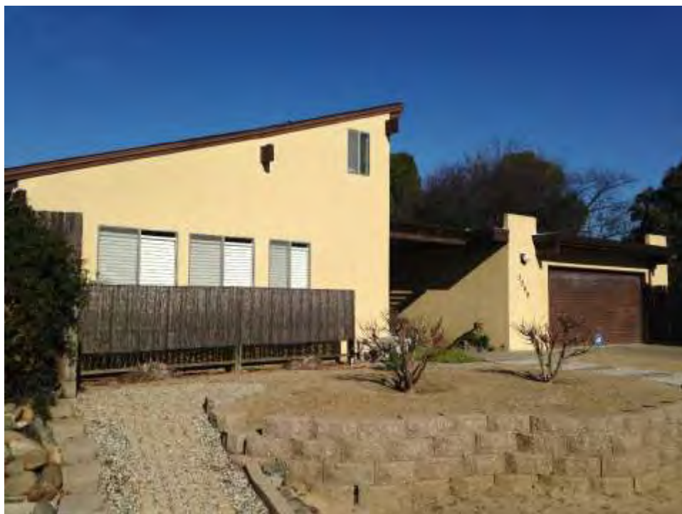
Photograph 6: Moderately altered Shed houses at 2208 Anza Avenue, 1972.
