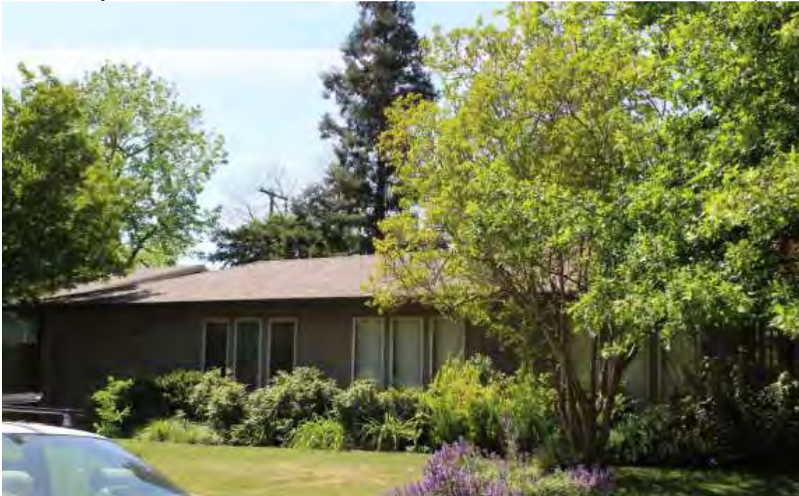
Photograph 11: 642 Elmwood Drive, east elevation, Streng Brothers, 1959.
