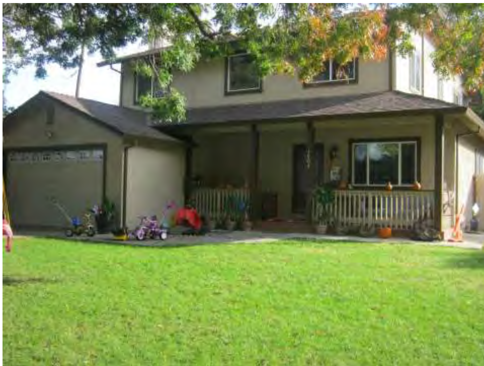
Photograph 12: Heavily altered house at 1603 Cypress Lane, 1962.
