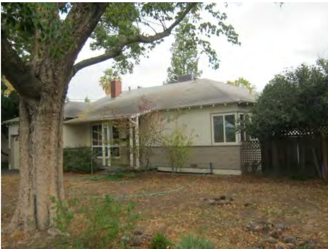
Photograph 10: 712 Hunt Way, Example of moderately altered Minimal Traditional house with hipped roof, 1952.
