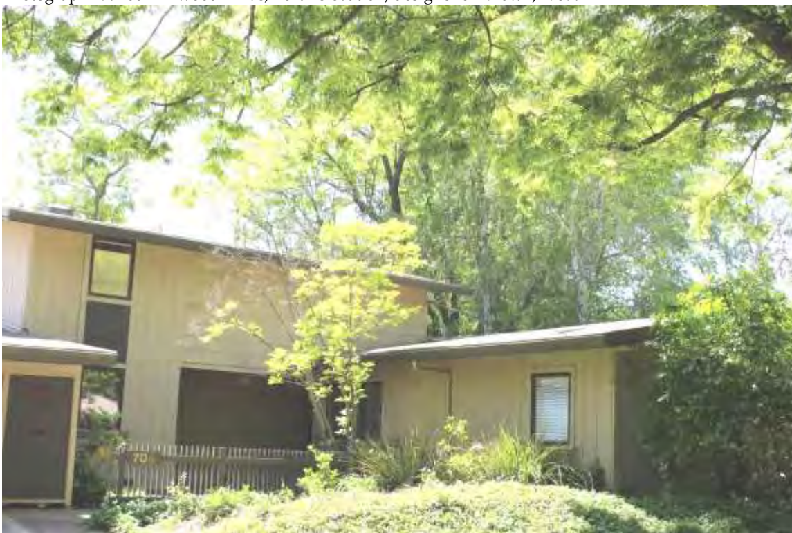
Photograph 20: 708 Elmwood Drive, north and east elevations, Dick Rohrbach/Gail Sosnick, 1958/1968.
