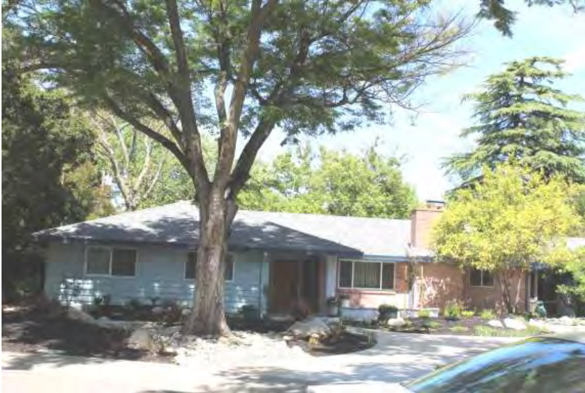
Photograph 23: 720 Elmwood Drive, south elevation, Dick Rohrbach, 1960.
