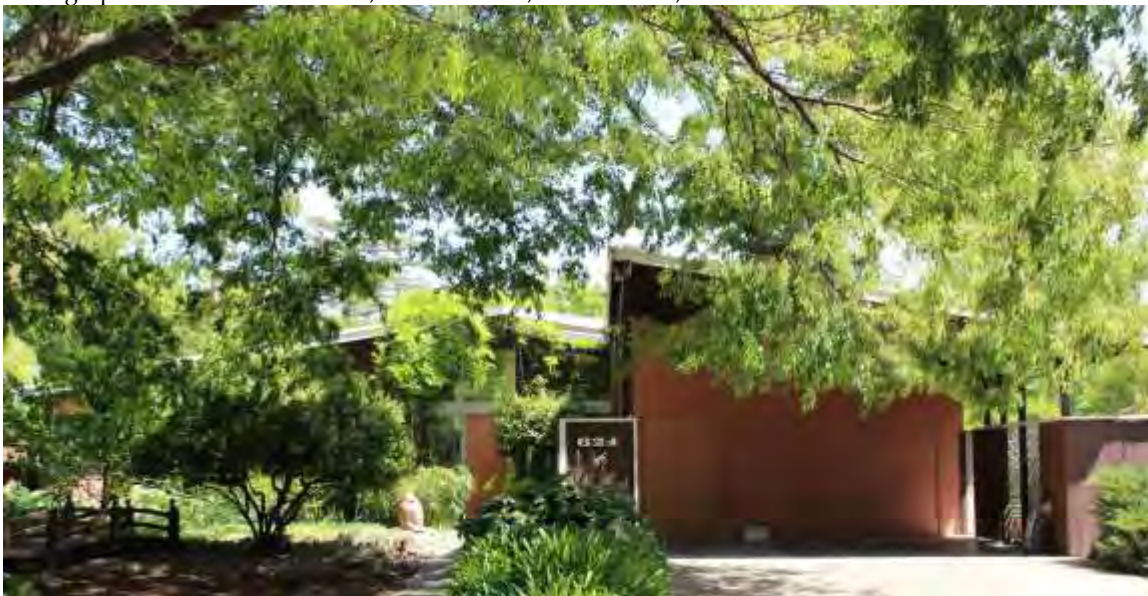
Photograph 4: 621 Elmwood Drive, west elevation, Gale Sosnick, 1959.
