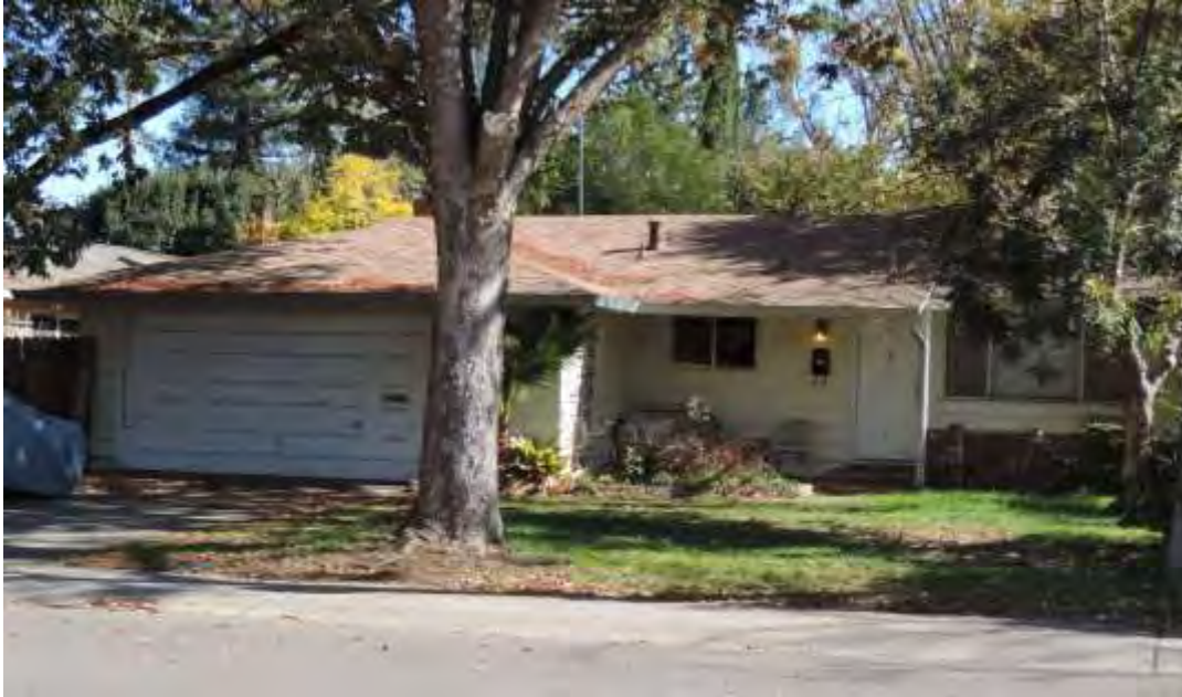
Photograph 4: 1108 Cypress Lane, Example of unaltered L-shaped Ranch house with hipped roof, original wooden garage door with decorative wooden trim, and original horizontal aluminum slider windows.
