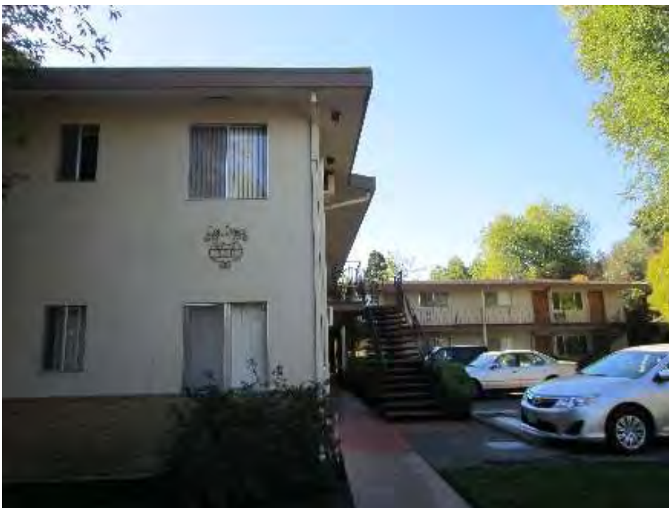
Photograph 6: 321 Ninth Street, Cal Davis Apartment, Garden Apartment, 1961.
