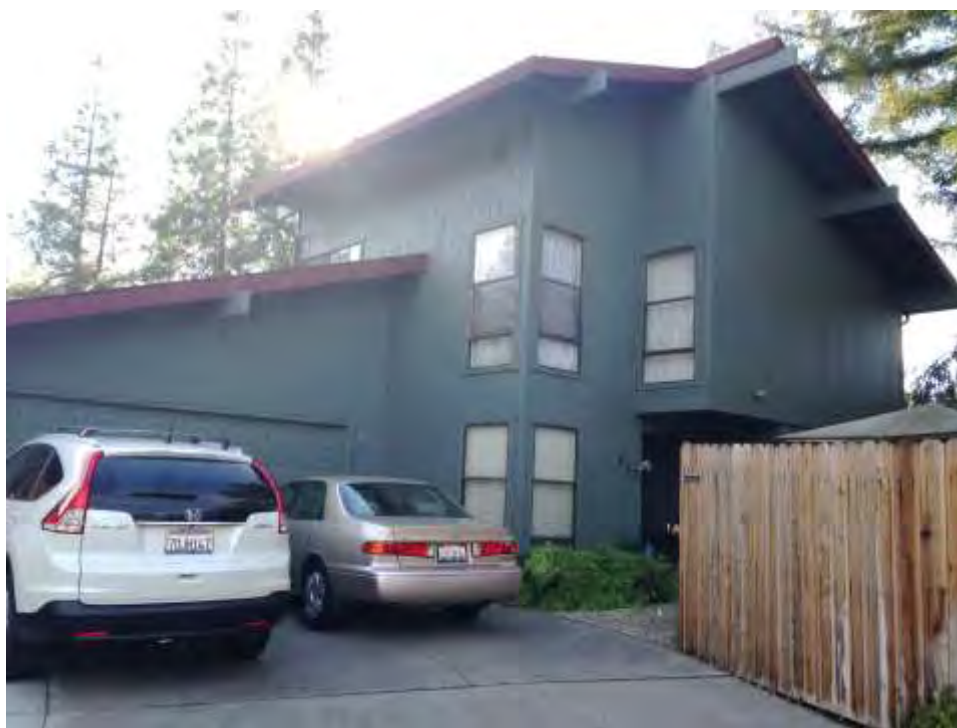
Photograph 14: Moderately altered 2-story Shed house at 652 Bianco Court, 1974.
