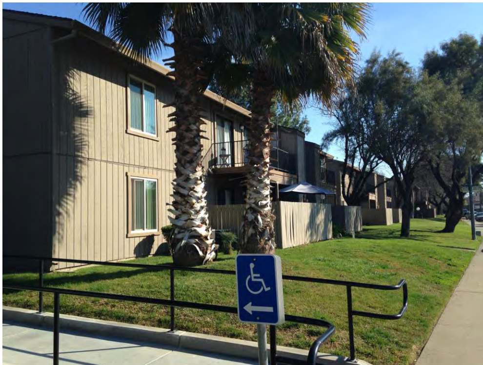
Photograph 1: 4735 Cowell Boulevard, El Macero Village, 2-story side-gabled apartment complex with second story balconies and iron railings, 1973.
