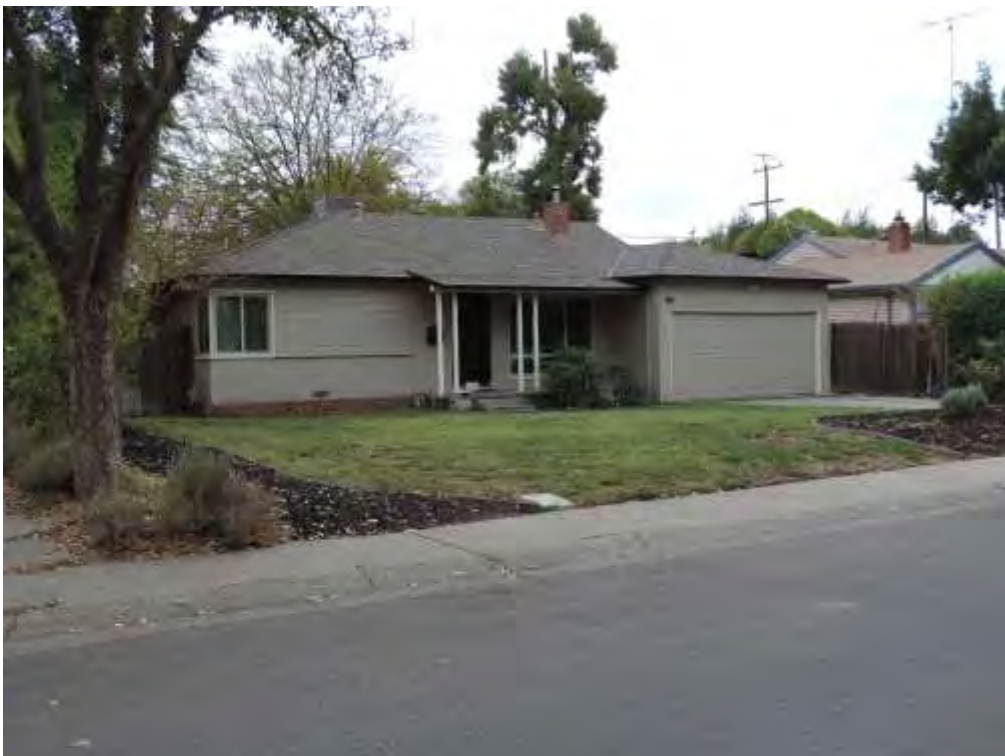
Photograph 2: 916 Pennsylvania Place, Example of moderately altered Minimal Traditional house with hipped roof, 1951.
