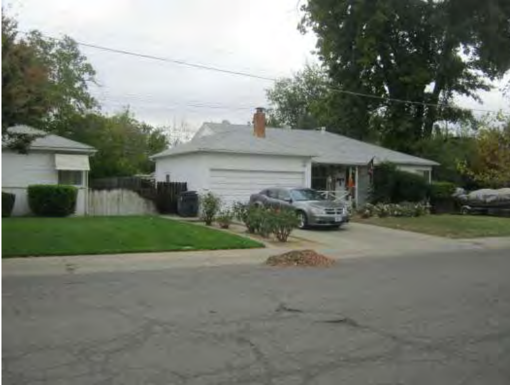
Photograph 9: 664 K Street, Example of unaltered Minimal Traditional house with hipped roof and two-car garage, 1951.
