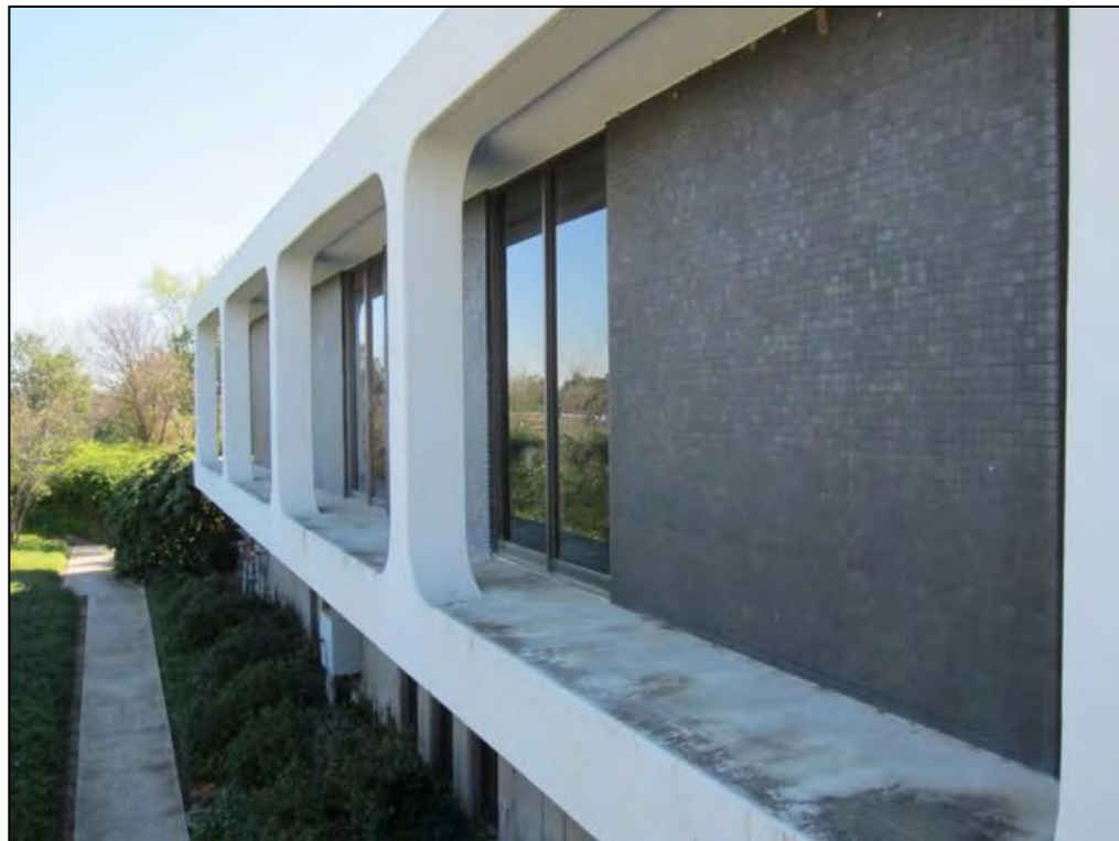
Figure 14: Photograph of colonnade on northeast façade, 1 March 2015.
