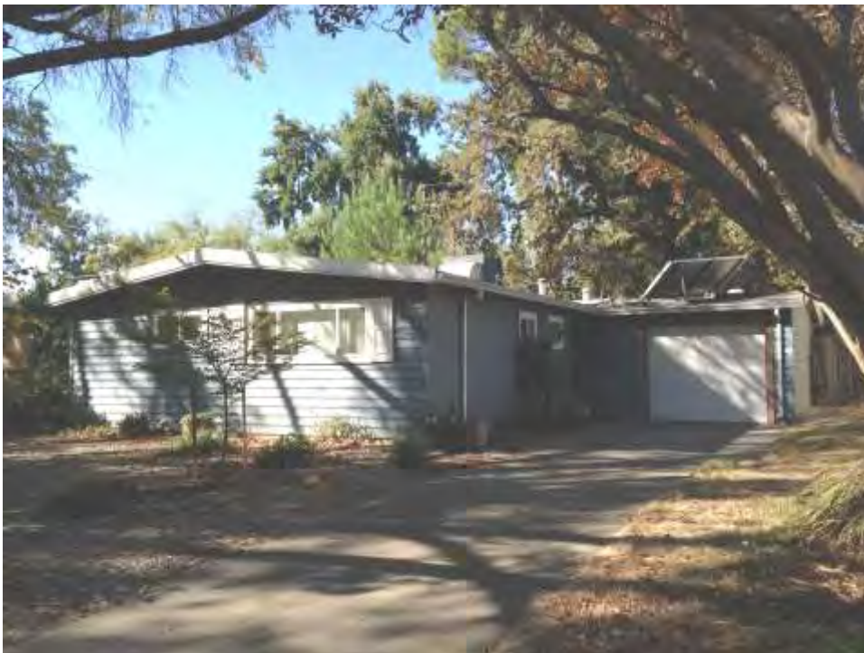
Photograph 3: Moderately altered house with membrane roof at 713 M Street, 1956.
