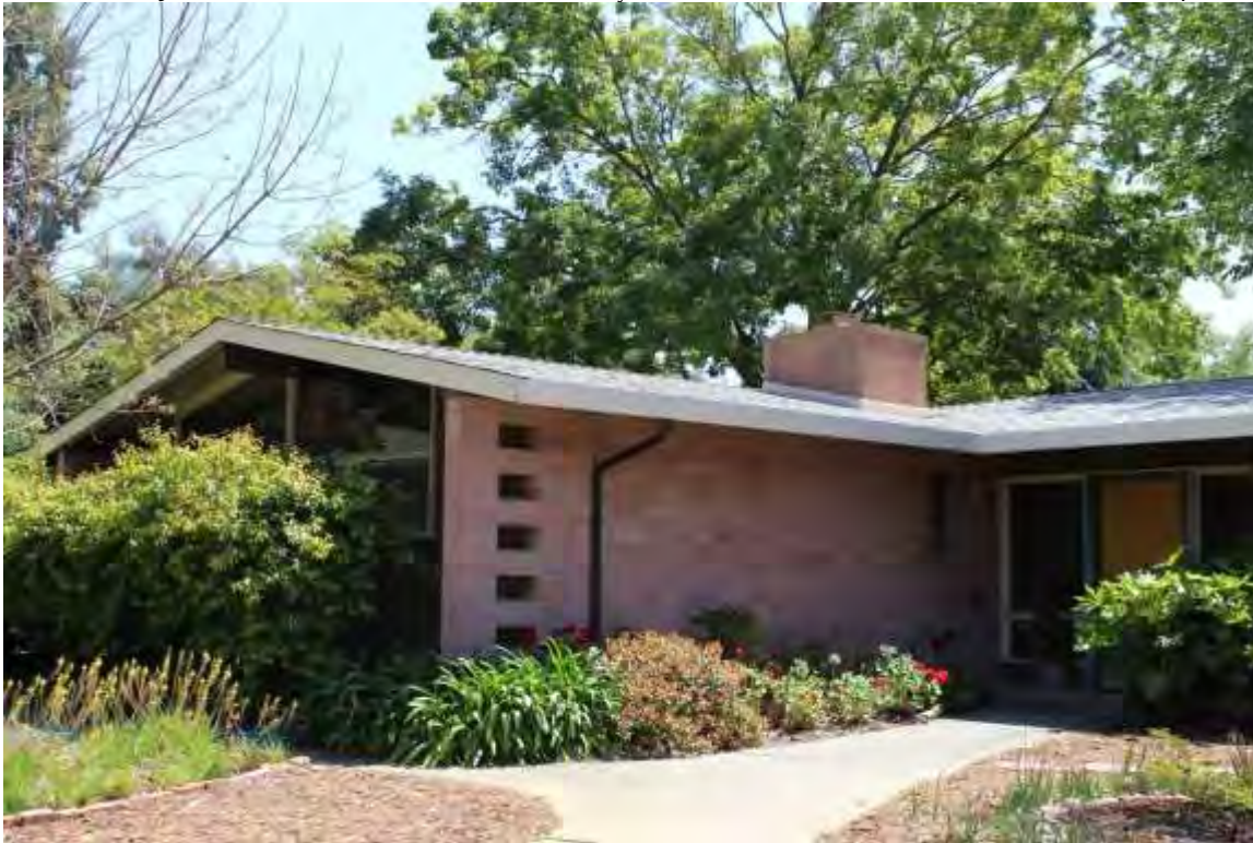
Photograph 31: 736 Elmwood Drive, northwest and southwest elevations, Dick Rohrback, 1959.
