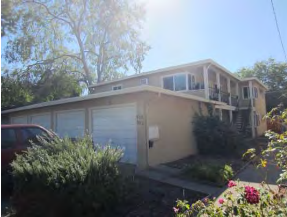
Photograph 1: 802 – 808 Tenth Street, Heavily altered two-story apartment building with ground-floor garages.
