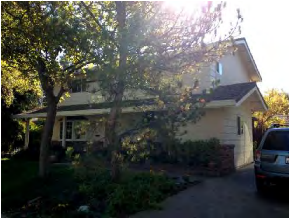
Photograph 5: 506 Citadel Drive, Example of moderately altered two-story house, 1969
