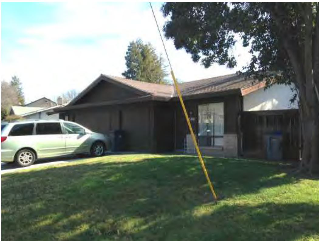
Photograph 4: 3960 Cowell Boulevard, Example of moderately altered linear duplex with cross gabled roof, 1973.
