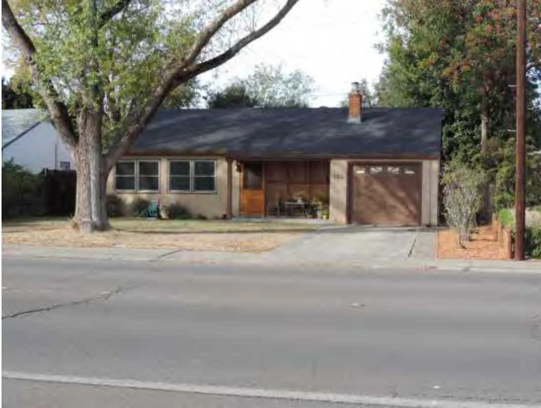
Photograph 2: 901 L Street, Example of lightly altered side-gabled Minimal Traditional house with multiple-light picture window, double-hung wood sash windows, and single garage with metal replacement door.
