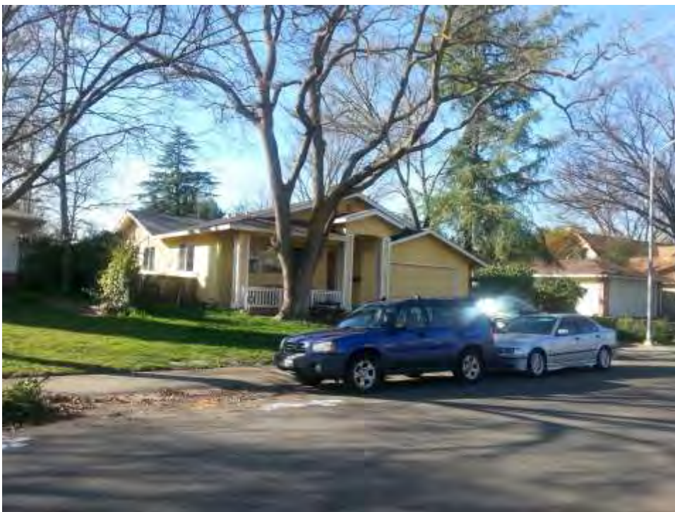
Photograph 15: Heavily altered house at 1331 Whittier Drive, 1966.
