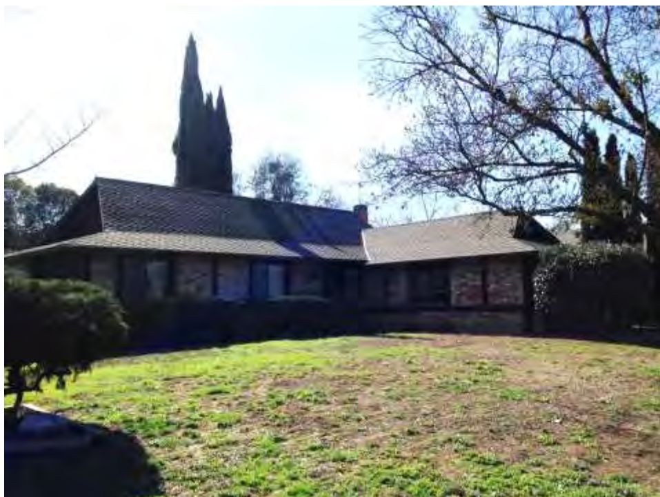
Photograph 2: 3730 El Segundo Avenue, Example of moderately altered L-shaped house with gable on hip roof, 1966.
