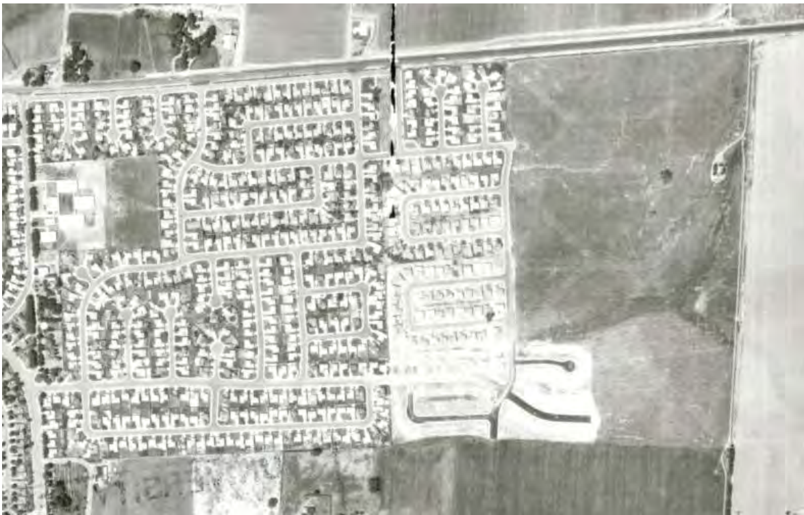
Figure 11: U.S.D.A. Aerial photo showing of Davis Manor 12, 13, and 14 complete with 15 under construction, 1971.
