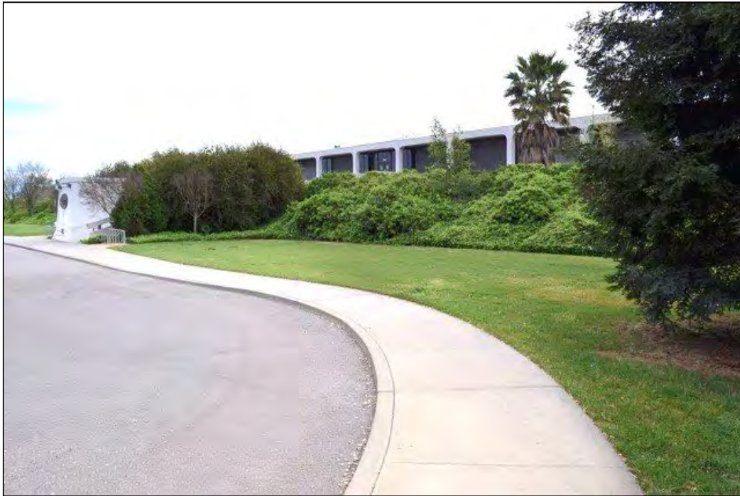
Figure 11: Photograph of northwest façade of building, camera facing southeast, 1 March 2015.
