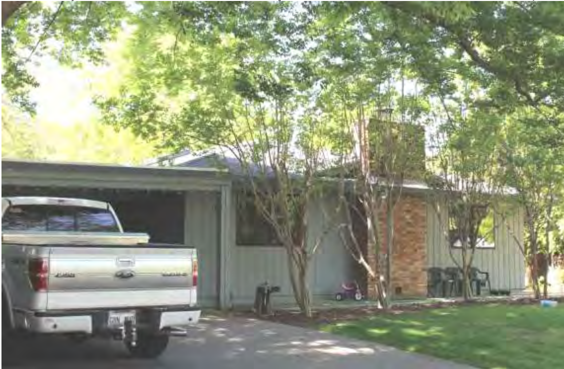
Photograph 35: 751 Elmwood Drive, east elevation, designer unknown, 1963.
