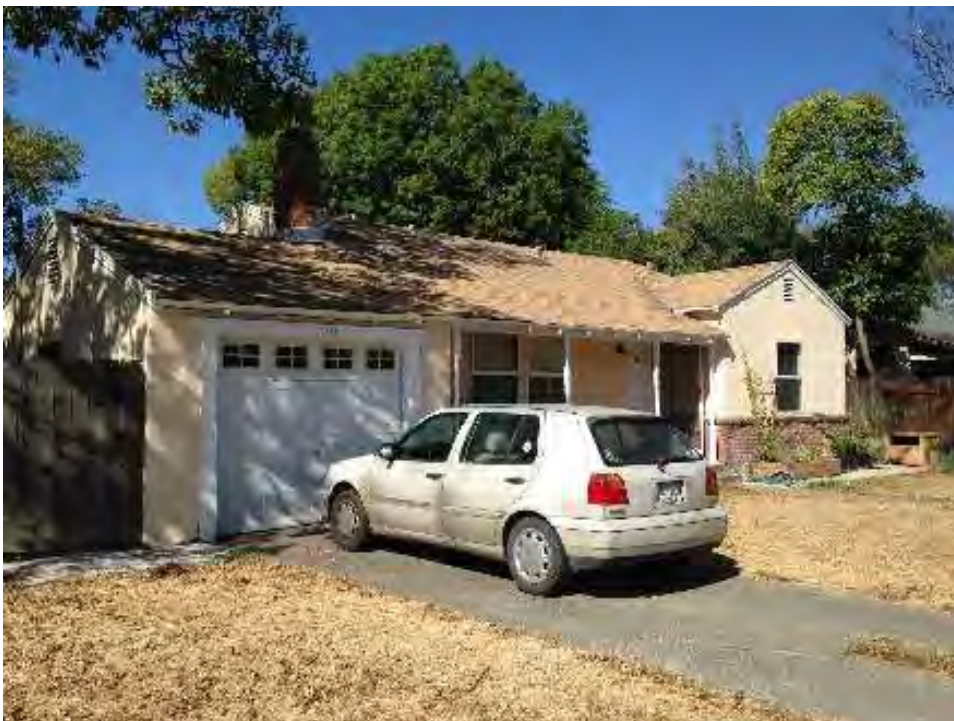
Photograph 2: 1101 H Street, moderately altered cross-gabled Minimal Traditional house with single garage.
