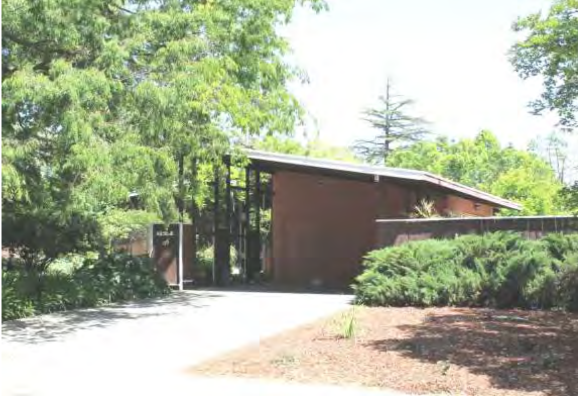
Photograph 5: 621 Elmwood Drive, west and north elevations showing projecting carport, Gale Sosnick, 1959.
